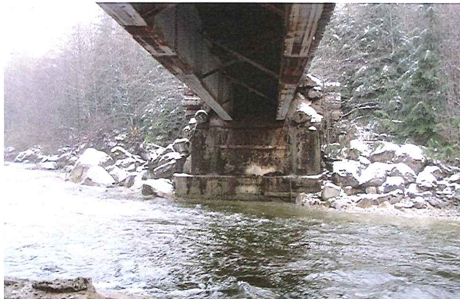
CK-2022 Abutment Left Bank
