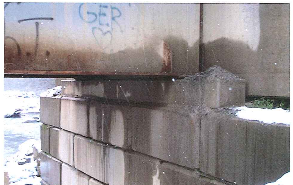
CK-2022 Abutment Right Bank 2
