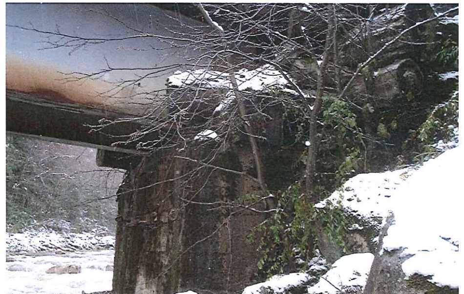
CK-2022 Abutment Left Bank 2
