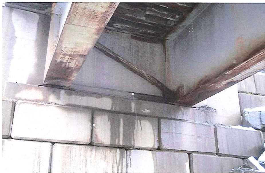
CK-2022 Abutment Right Bank
